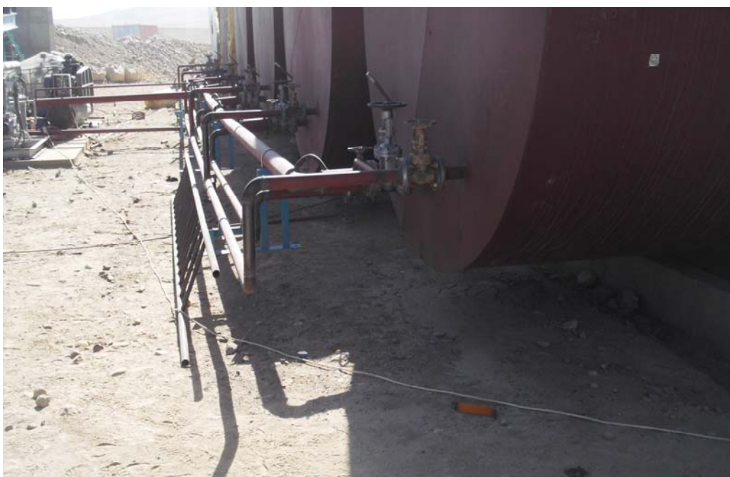
Photo No. 7: Bitumen reservoir without secondary containment
