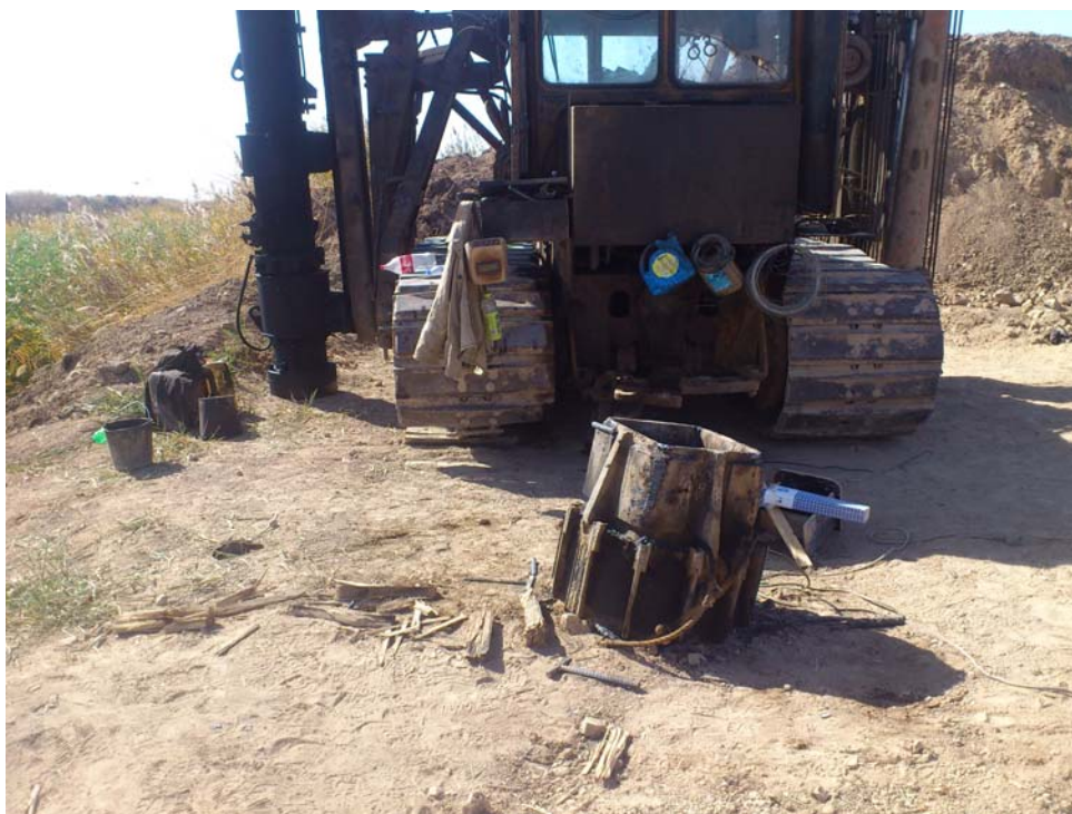
Photo No. 4: Improper handling of oil/lubricants
